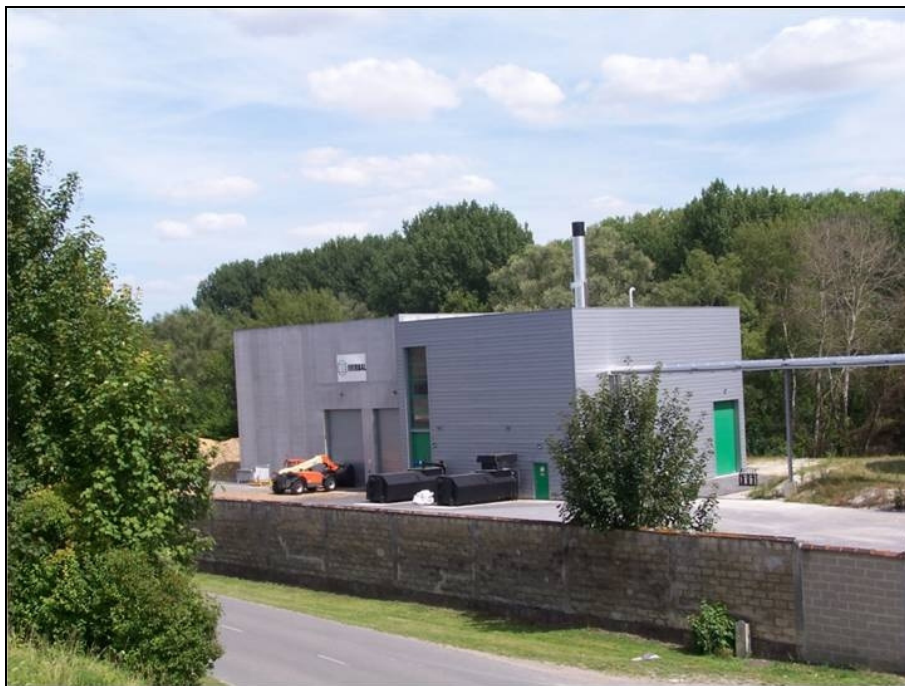
Building housing the biomass boiler - EVERBAL
