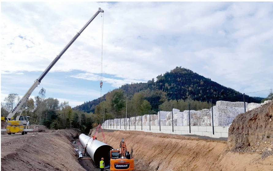
Papeteries de Clairefontaine – Installation of a retention system for firefighting water
